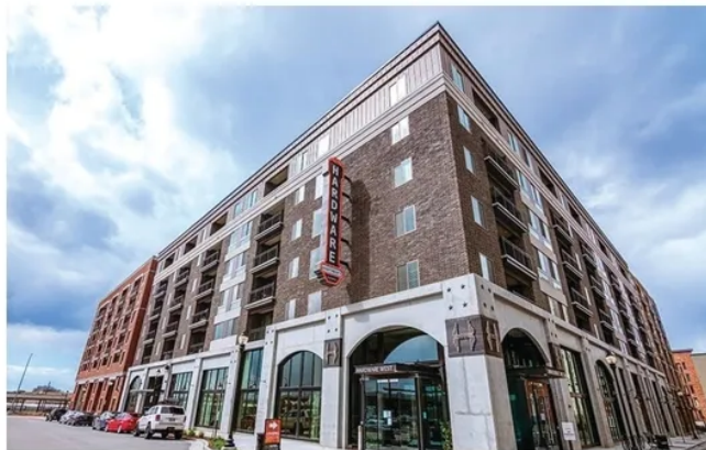
Hardware Village benefits from direct access to the TRAX light rail and FrontRunner commuter rail, connecting Salt Lake City with Ogden and Provo.
